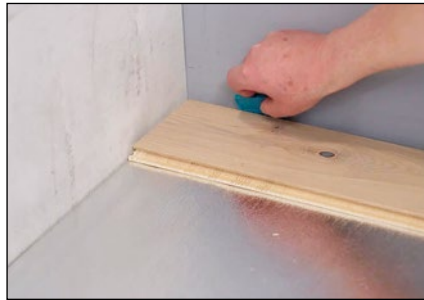
Centre/angle the installation area and adjust the first row of planks by cutting it to size.
